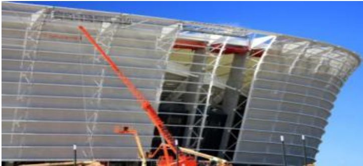
• Greenpoint Stadium CT
